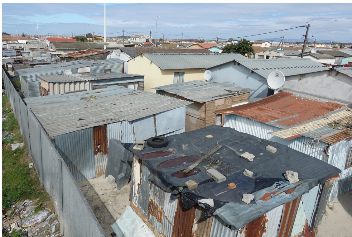
Figure 2. Shacks built in the backyard of RDP houses (photo by Arno Suzuki, 22 August, 2018)
